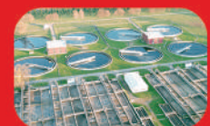
Environmental Engineering and Wastewater Treatment
